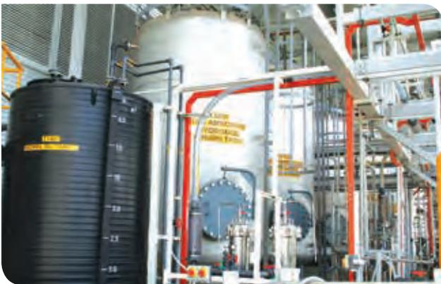
its overall system as pilot plant scale test units in application for different industries. With this, the Group has positioned themselves as a first mover within the application of the Aquaporin Inside(tm) Forward Osmosis technology and have pre-knowledge on ZLD wastewater treatment operations and applications.
